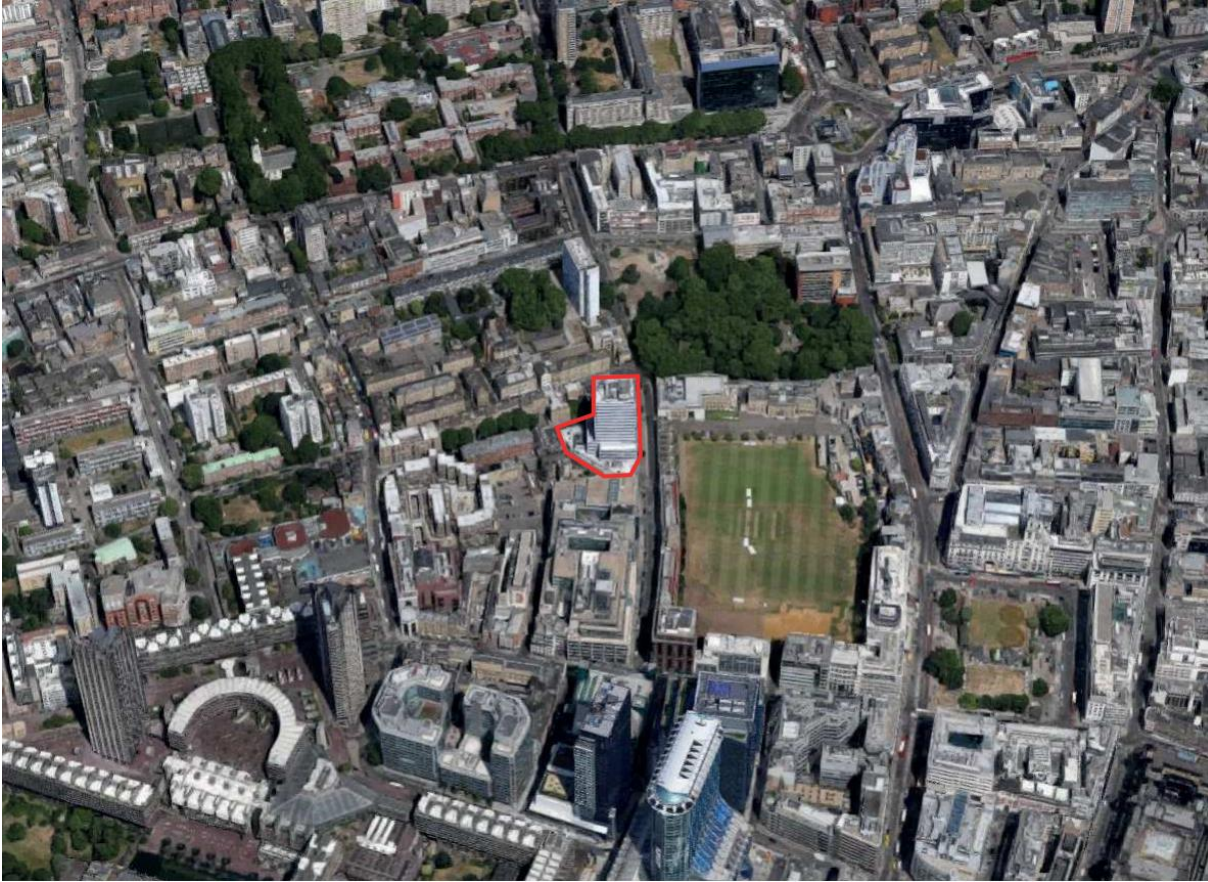
Aerial view of site from the west
