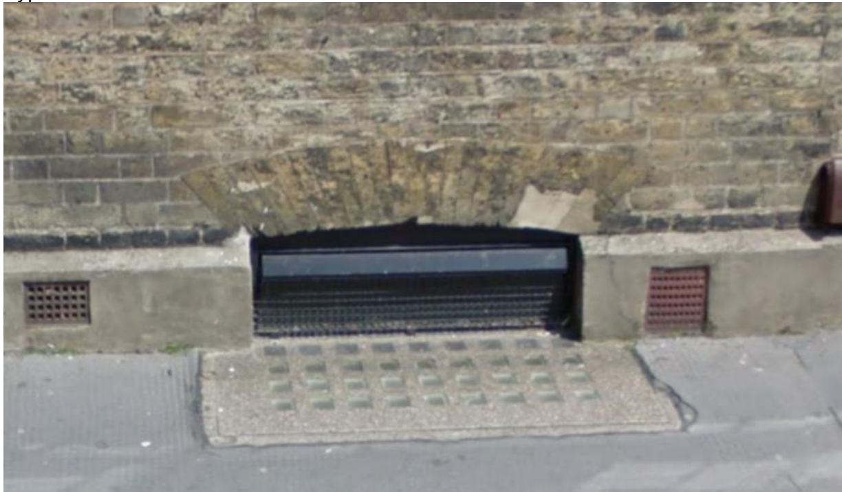
Typical basement window at No. 25 Bunhill Row
